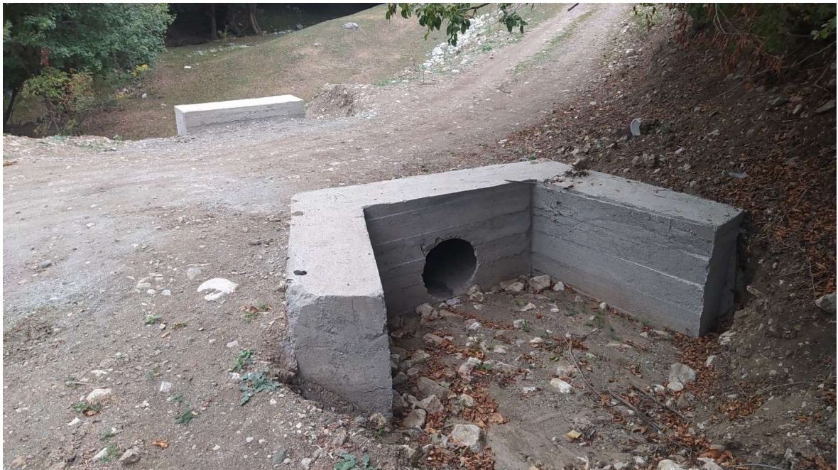
Repaired field roads
