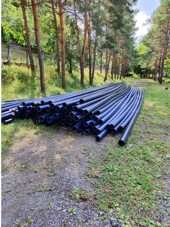
Pipes for irrigation network construction
